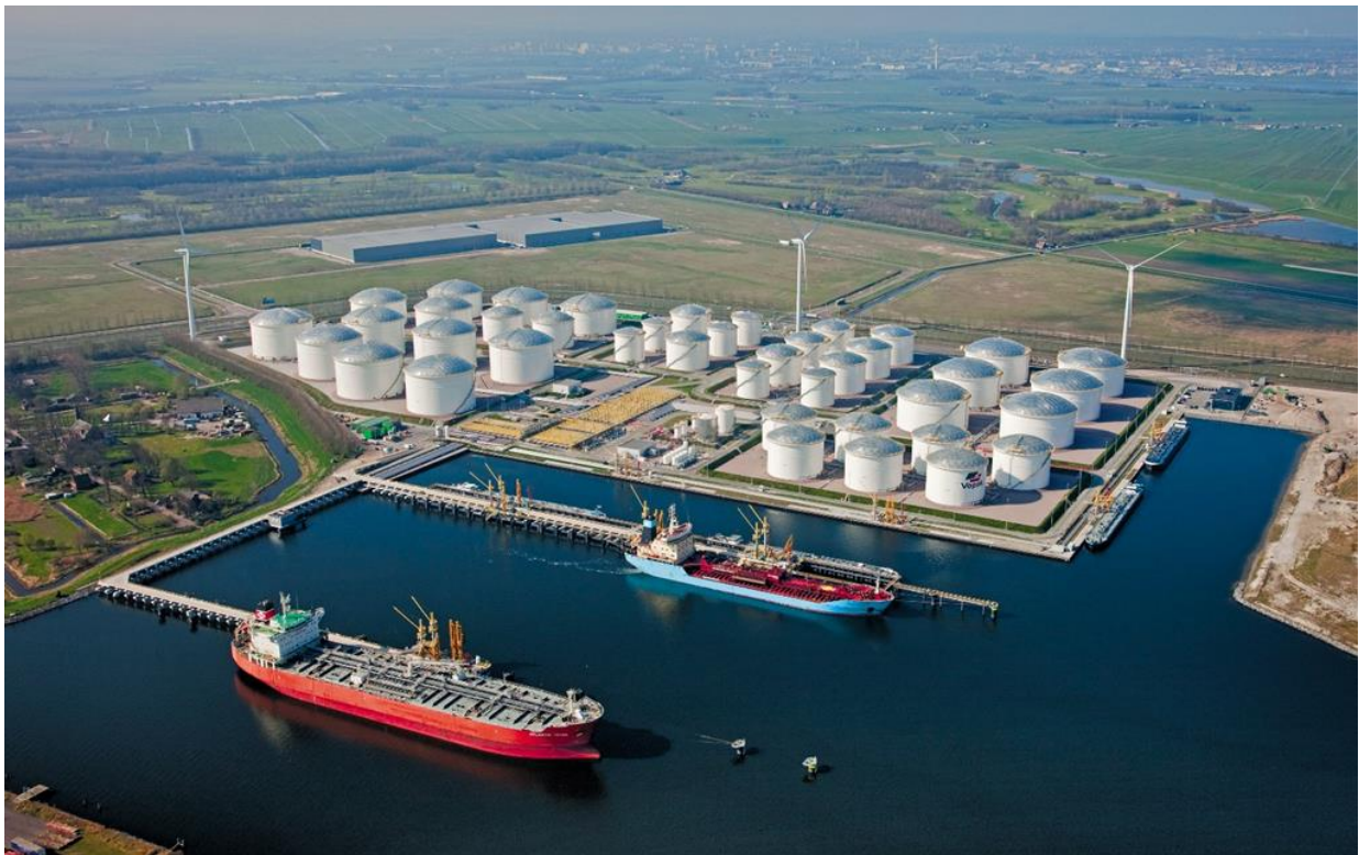
Figure 3: Tank farm with ship loading and unloading area
